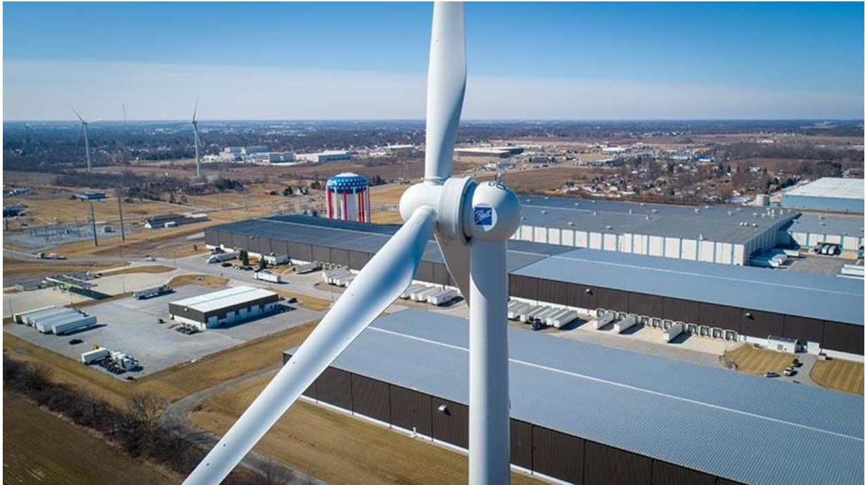
A megawatt-class turbine in a behind-the-meter distributed wind application. Photo by Hank Doster, One Energy Enterprises LLC
